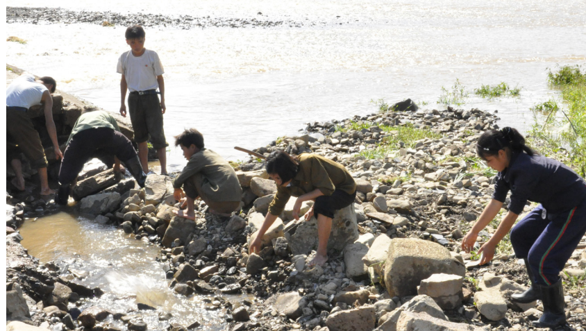
Local people engaged in road repair after flooding.
