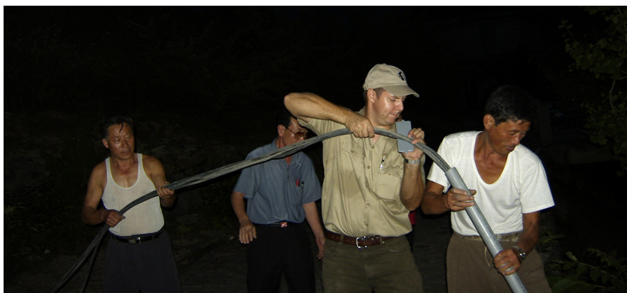
Pulling the cable to connect the generator.
