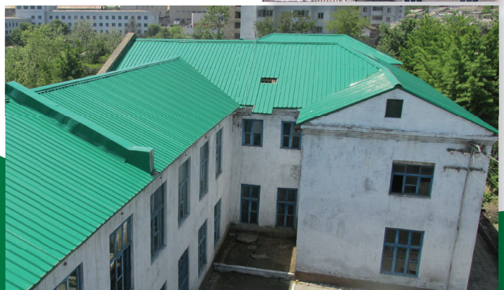
New roofing installed at Pyongyang #2 Hepatitis Hospital.
